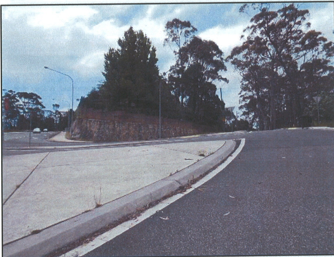
Corner of Great Western Highway and Queens Road – view west
